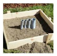
Backfill the hole being careful not to get too much dirt in the sweeps.
