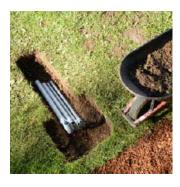
It's always a good idea to set your preassembled sweeps into the hole to make sure they will all fit and are long enough to clear the new concrete slabs perimeter.
