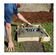
After your concrete is mixed and the form is filled with concrete, use a trough to smooth out the concrete evenly. Sloping the concrete slab slightly will assist in keeping water from pooling around the bottom of the pedestal.
