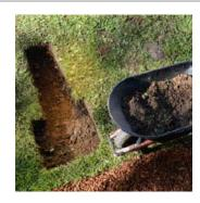
Once you locate a good location, dig a hole in the pictured shape to account for your conduit sweeps and concrete slab.
