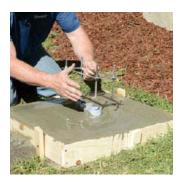
Before the concrete cures completely, install the pedestal-mounting template by pressing the 4 L-bolts down into the concrete until 2" of each bolt is still visible. Slightly moving the template back and forth will help with air bubbles and insure the template sits flat.
